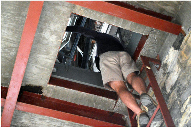
Mark Babcock climbs up the ladder to the bell chamber.
