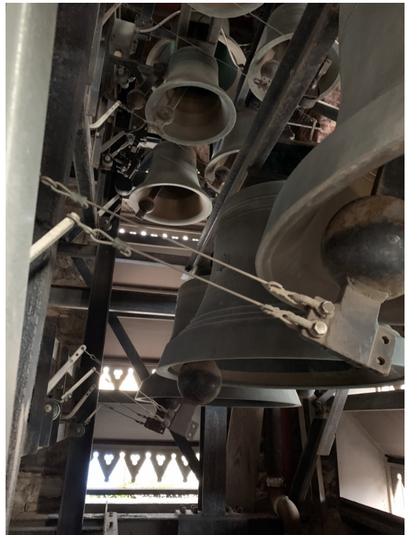
Unlike a piano keyboard, the bells are not arranged in chromatic order. Big bells are mixed with small bells in order to fit
